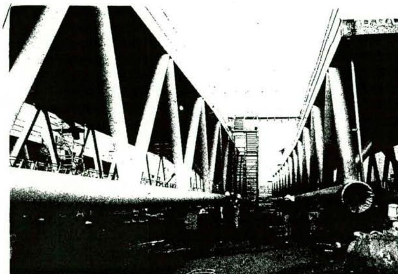
Fig. 5: Bridge elements 105 m long at fabrication yard
