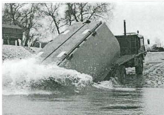
The anchorage points are released and a centre bridge section slides off the lorry into the water.
