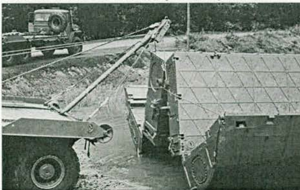
Hook up and folding of a centre section. Visible difference: different construction of the crane and of the loading and unloading equipment.
