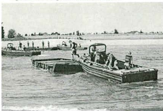
The bridge in position. The first vehicles roll on while the tugboats hold the bridge in position against the current.
