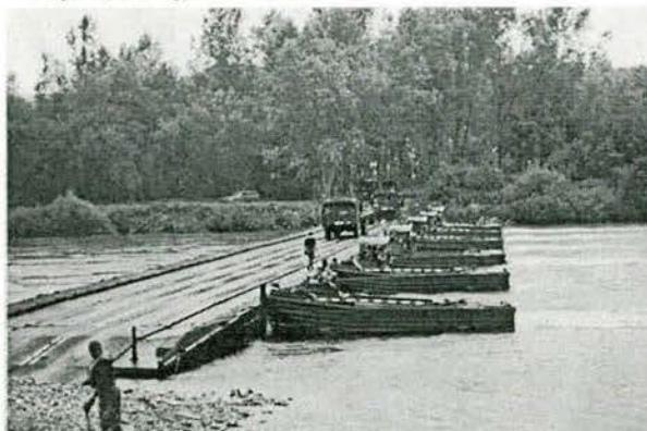
The bridge in position. The first vehicles roll on while the tugboats hold the bridge in position against the current.
