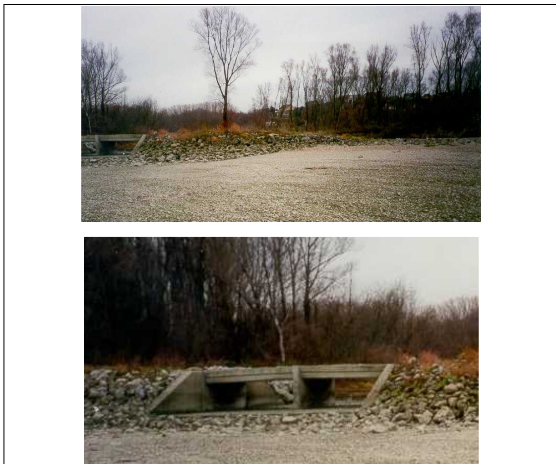
Figure 3.6. Engineering measures to improve the hydrological connectivity, a) lowering the riverside embankments, b) artificial openings at inflow channels (photos: Verheijen).
