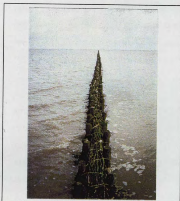
Fig. 4.4: Wave reduction by a brushwood groyne.
