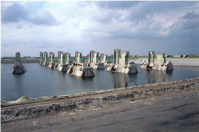
Serial construction of piers.
