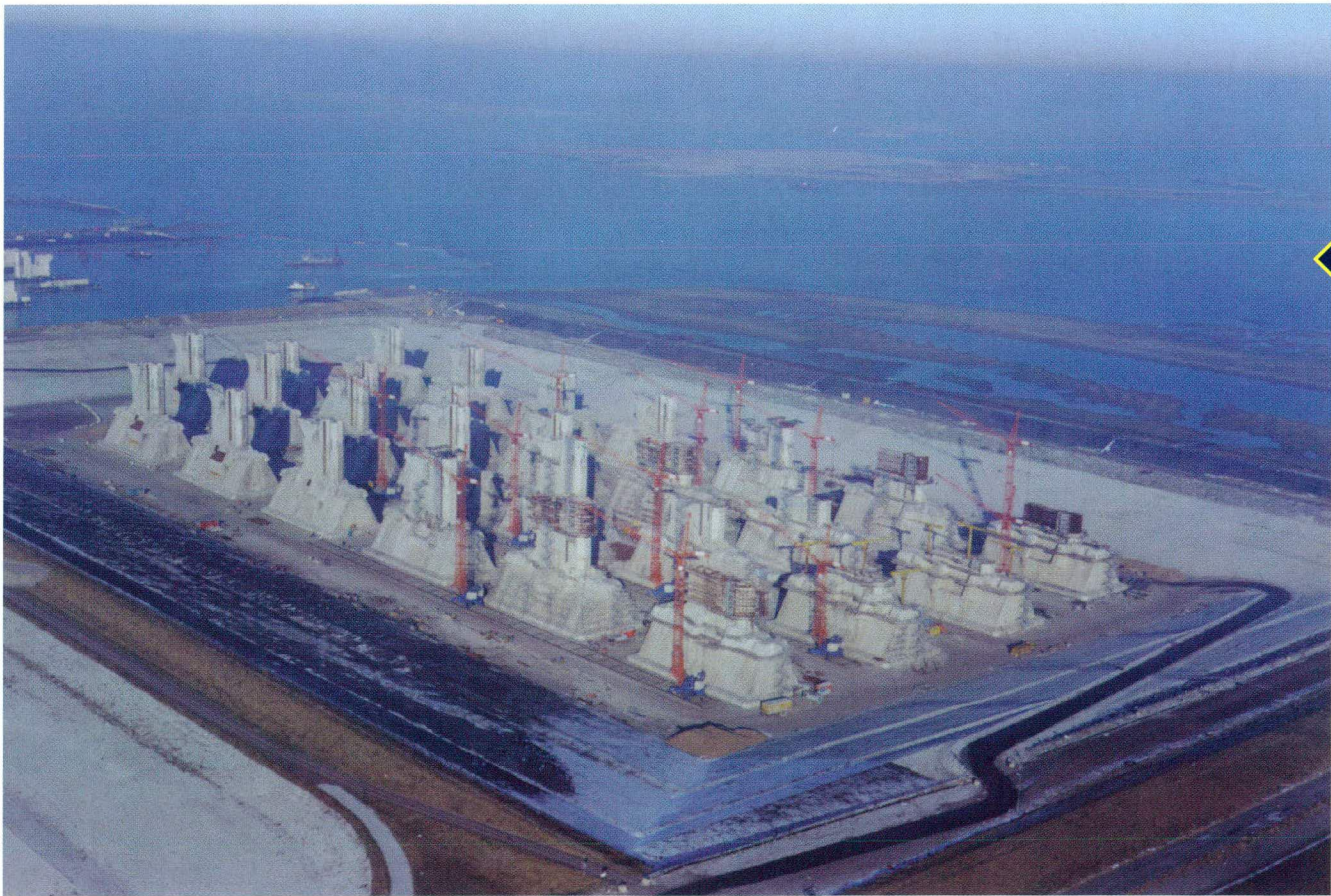
Serial construction of piers.
