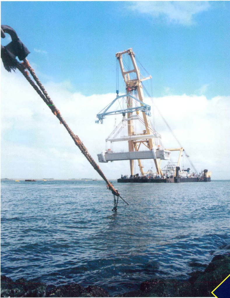
The Taklift IV crane vessel with a road bridge box girder in its hoist.
