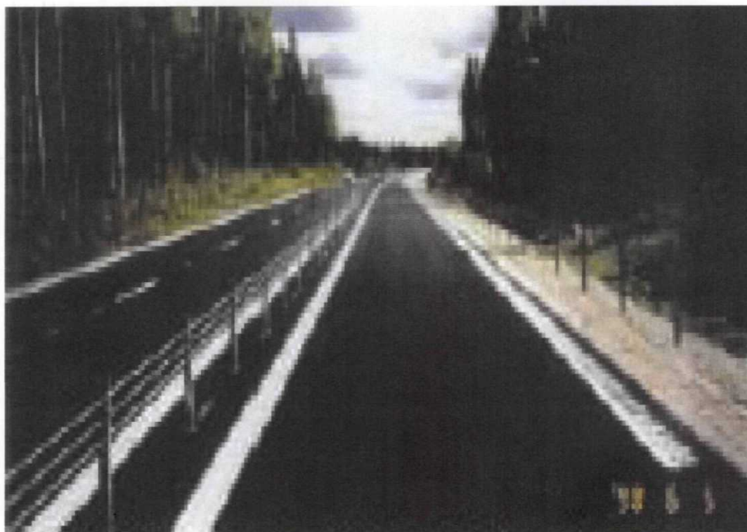
FIGURE 6 Example of side cable fence in a forest area.
